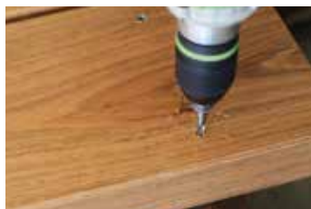
Step 1: Pre-drill with SPAX step drill 6mm diameter over the entire screw length (see page 92). The wooden decking board displayed is 45mm thick.
